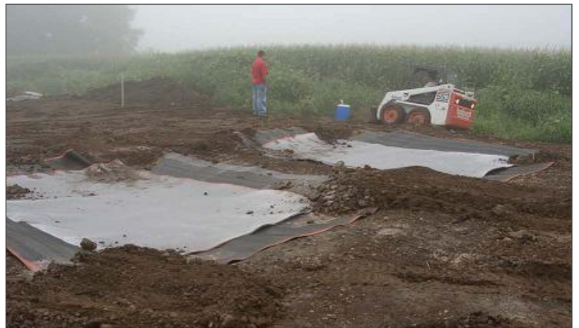
Figure 4: Construction of pan lysimeters similar to those used at the site.
