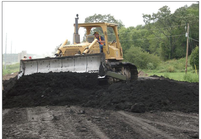
Figure 1: Spreading the foundry sand with a bulldozer.
