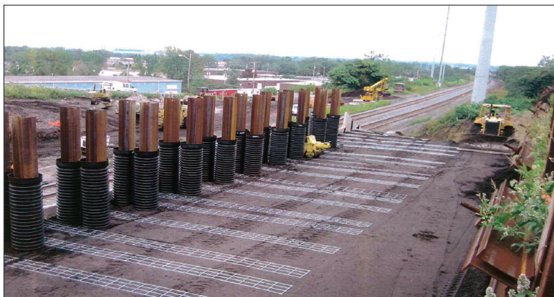
Figure 1: Compacted foundry sand behind MSE wall.
